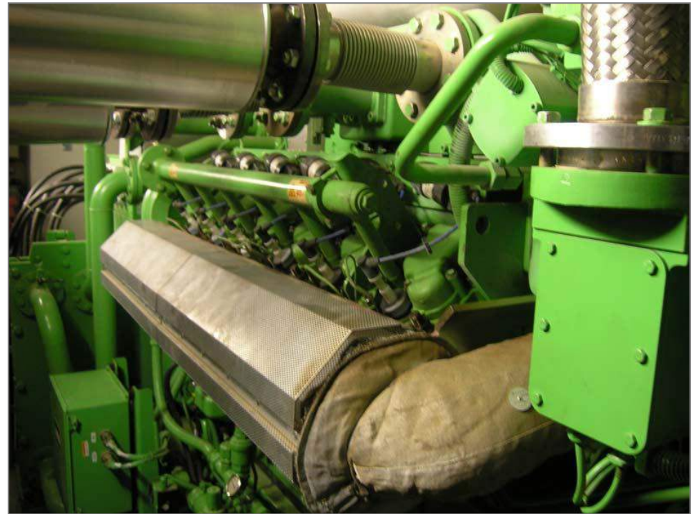
CHP 100 KW, usage of thermal energy for apartment and drying of grains, GRENOL GmbH
